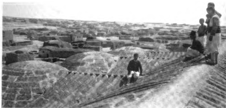
Fig. 4. View of Misti from the roof of the Church.
